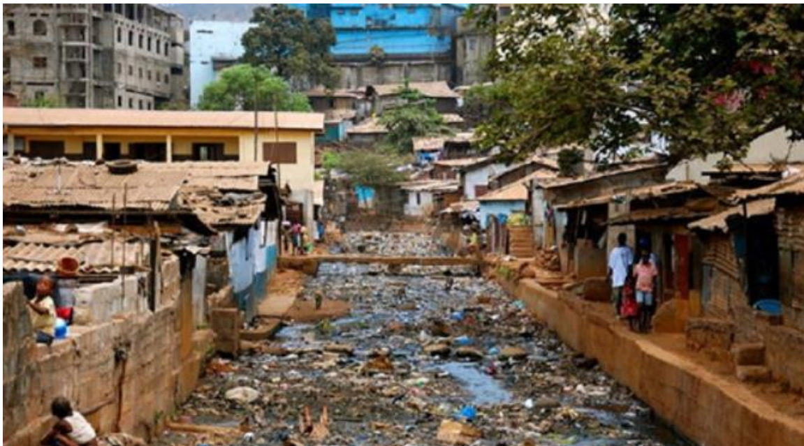
Figure 6: Urban Decay and Environmental Degradation in an Informal Settlement in Abuja.
